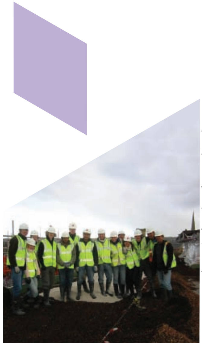
Sharrow Primary School, by Sheffield Design and Project Management, Sheffield City Council © Cath Basilio
